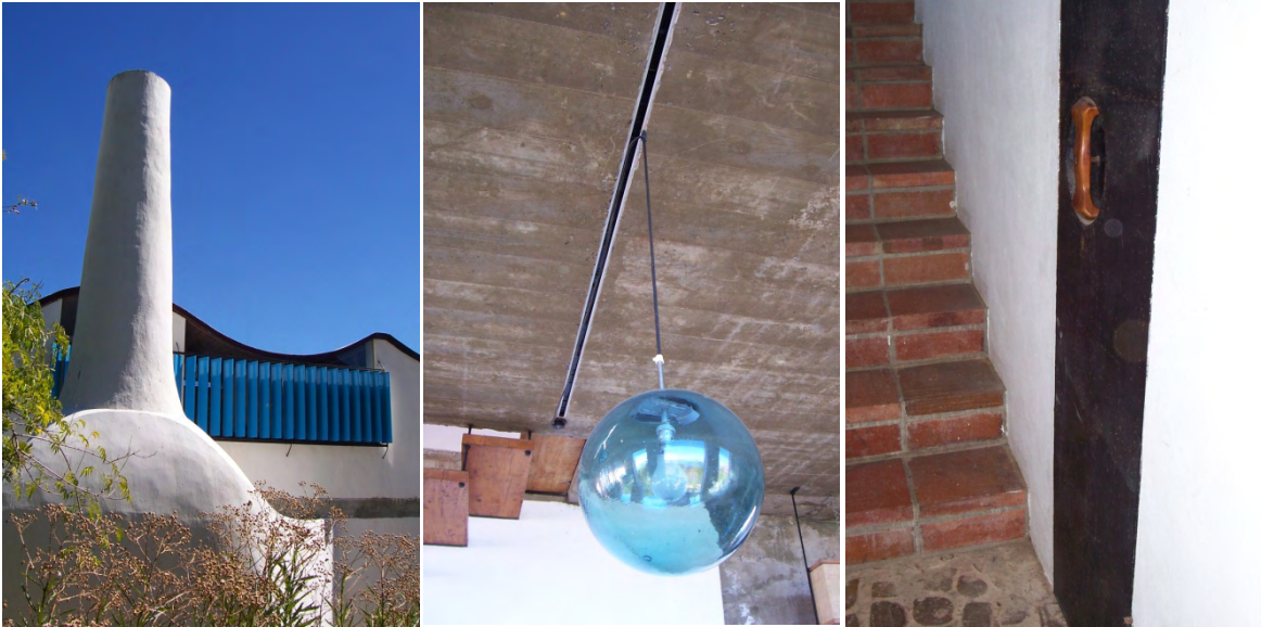
Figure 7.41. Die Es (1965): Chimney; in-situ concrete first floor, timber treads and Japanese fishing buoy as lamp; quarry tile stairs leading to basement (Photo's courtesy of Auret, 2006).
