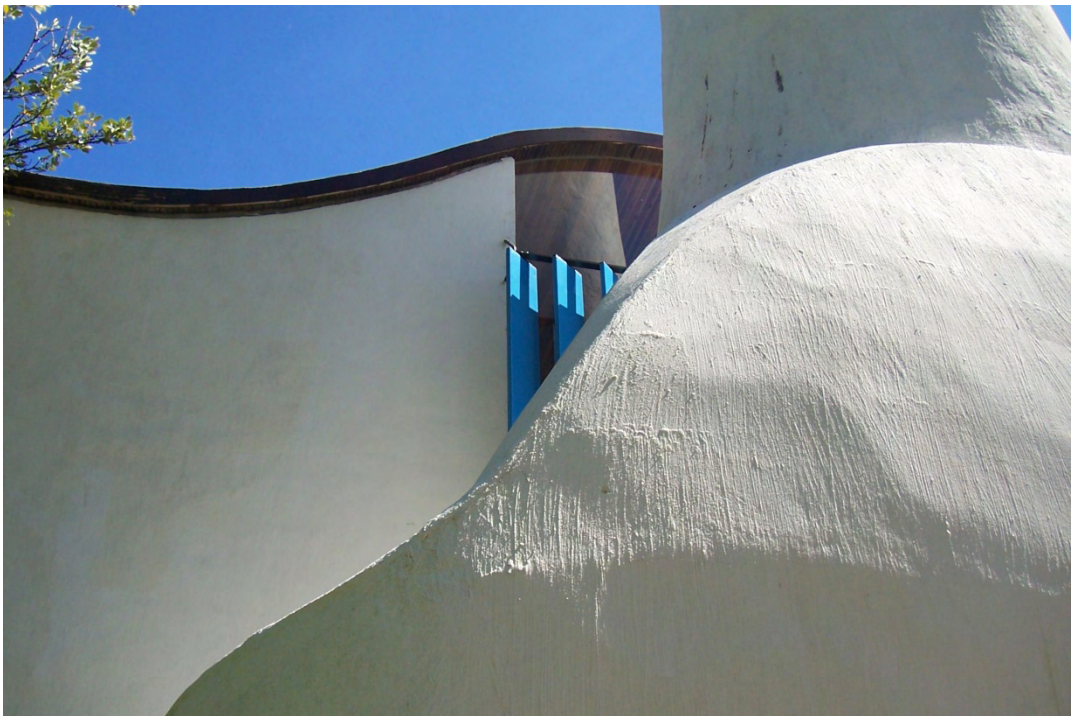
Figure 7.44. View of Die Es (1965) chimney showing plasticity of finish and form (Photo courtesy of Auret, 2006).
