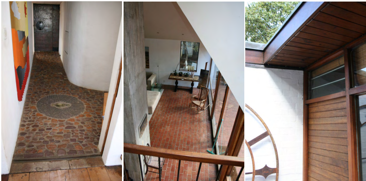
Figure 7.33. From the left: Stone pebbles as floor at Die Es (1965); brick floors at House Raynham (1967) and timber windows, door and eaves at House Raynham (All Author, 2008).
