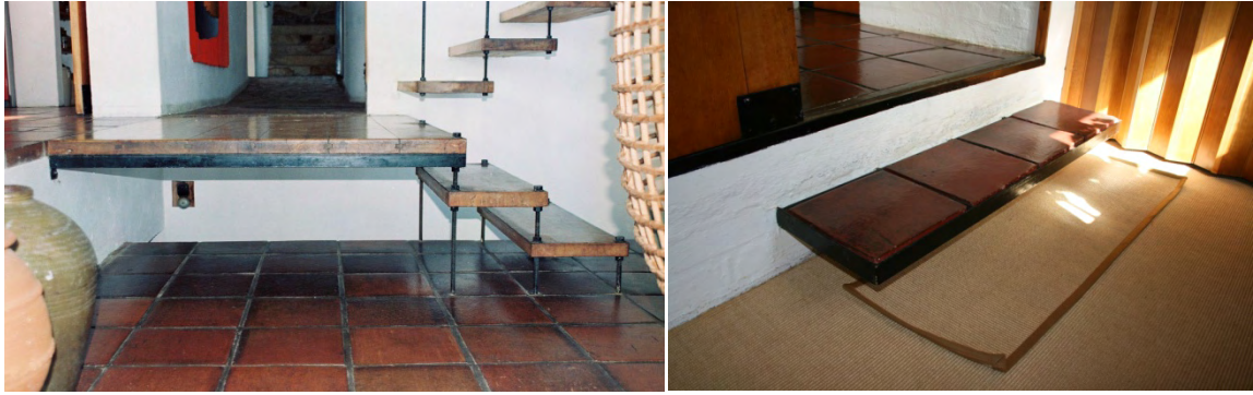
Figure 7.1. Left: Steel framed timber platform at the junction of living and entrance hall at Die Es (1965) (Fagan, 2012b). Right: Similar platform at junction between passage and main bedroom at House Keurbos (1951) (Author, 2008).
