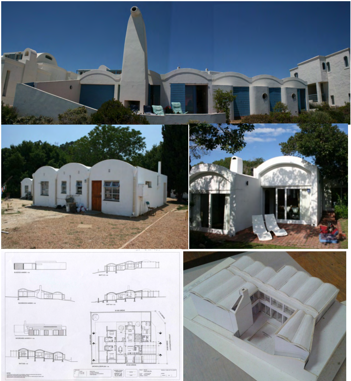
Figure 7.11. Top: Barrel vaulted roof at House Paradys (2003) (Author, 2009). Middle left: Barrel vaulted roofs to Idas Valley (1975) (Author, 2009). Middle right: House Lückhoff (1981) (Author, 2009). Bottom left: Proposed house with barrel vaults and linking mono pitch roofs to House Van Zyl (2007) (Fagan archive - Job No. 0702 24/03/2006). Bottom right: Model of House Visser (Author, 2012).
