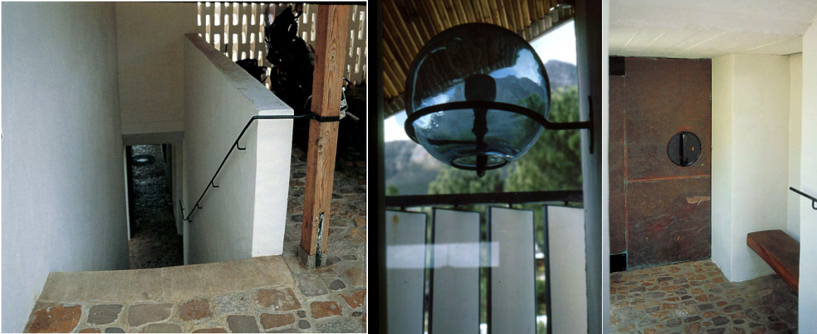
Figure 7.35. Left: Continuous steel rod handrail at Die E (Fagan, 2012b). Middle: Glass Japanese fishing float reused as light fitting at Die Es (Fagan slide archive, undated). Right: Front door at Die Es made from old copper boilers (Fagan, 2012b).
