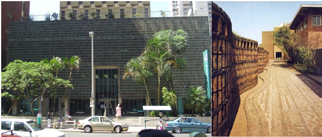
Figure 4.17. Left: The ceramic screen of Eaton's Netherlands bank in Durban 1961-5 (Author, 2004). Right: Eaton's woven brick wall at the Little Theatre in Pretoria (c.1950) (Harrop-Allin, 1975:97).
