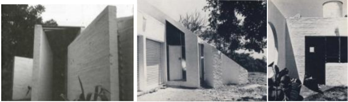
Figure 3.16. Previous page left: Anderssen House (1949), Pretoria, Norman Eaton architect (UIA International, 1985:22). Previous page right: House Biermann (1962) Barrie Biermann architect. Left: House Mikula (1965-7), Paul Mikula architect (Architecture SA, May/June 2005:14). Right: House Manor Gardens, Durban (1973) Hallen and Theron (Architect and Builder, February 1973:34-35).
