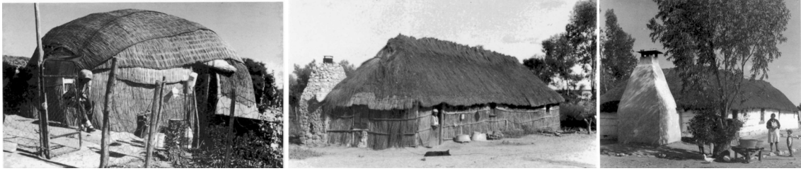
Figure 2.10. Progression of framed and reed structures. Left: A circular matjieshuis , Ou Tuin, Kamiesberg (Walton, 1997:18). Middle: Rectangular reed-walled cottage, Oudekraal Fontein (Walton, 1997:30). Right: L-plan reed-walled cottage, Oudekraal Fontein (Walton, 1997:31).
