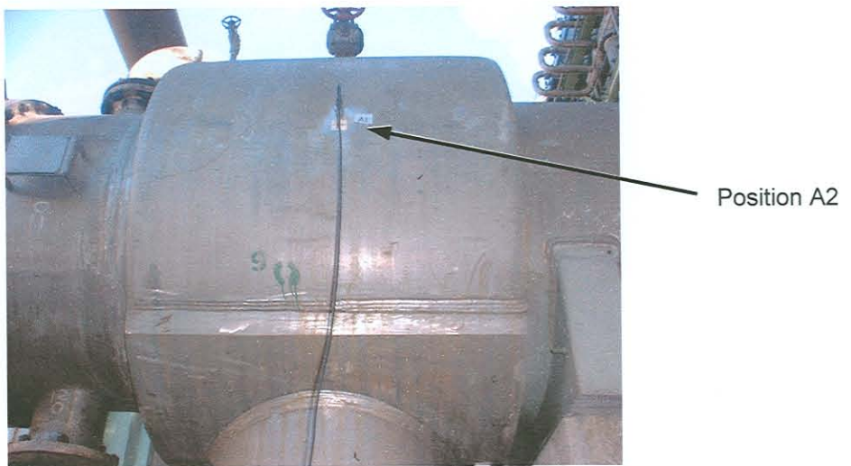
Figure D.5: Shell measuring position (A2) 90° from outlet
