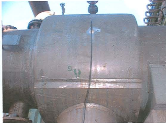
a) Measuring position at inlet of heat exchanger (A4) b) Measuring position 90° to outlet (A2) (Position 1 from figure 4.2)
