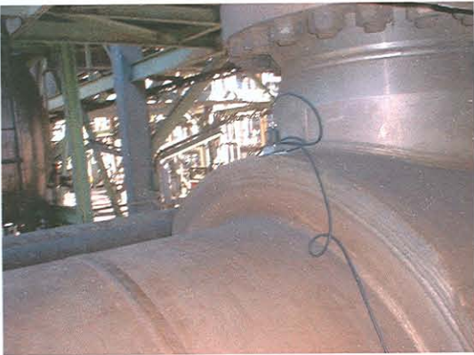
a) Measuring position at inlet of heat exchanger (A4) b) Measuring position 90° to outlet (A2) (Position 1 from figure 4.2)
