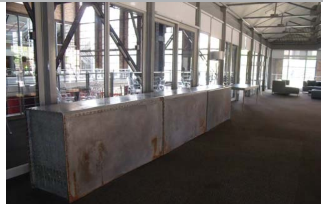
Fig.301:New glass partitioning with aluminium frames. [Source: author]
