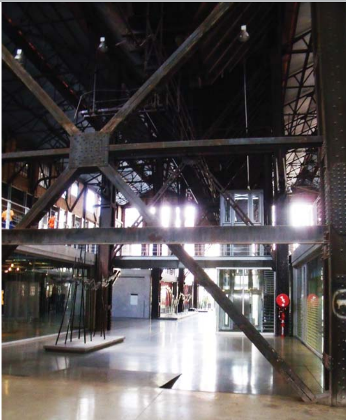
Fig.300:Existing steel bunker. [Source: author]
