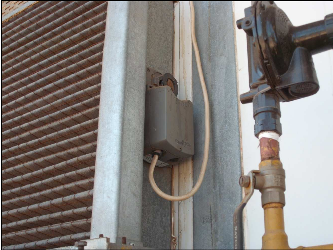
Figure 4-2 Actuator controlling inlet vent
