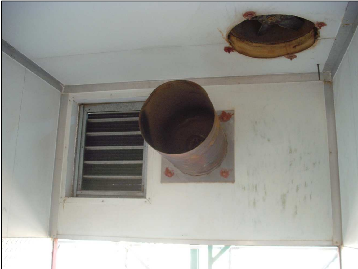
Figure 4-13 Gas burner, inlet vent and outlet fan
