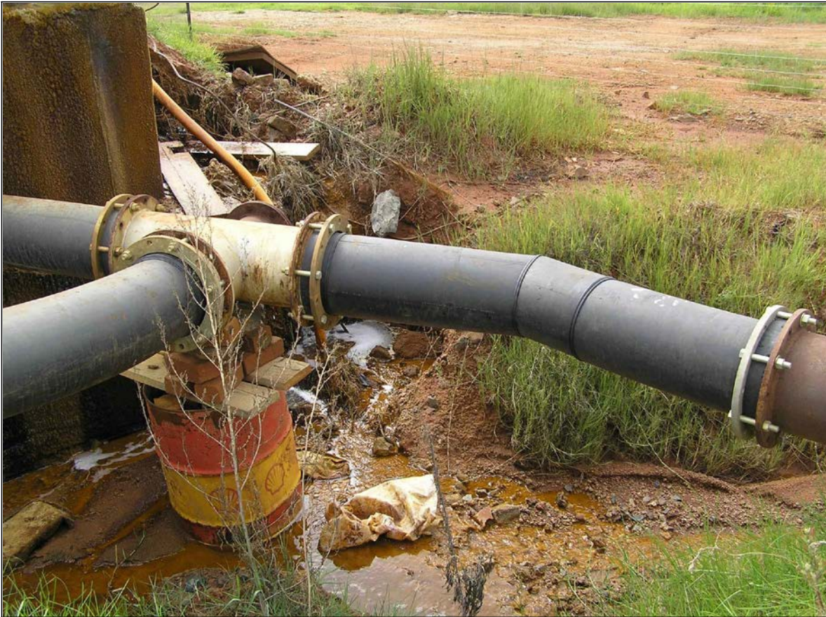
Figure 45: A disused Shell drum prevents a system of pipes from collapsing, Harmony Gold treatment plant, Randfontein, 2008. Photograph by the artist.
