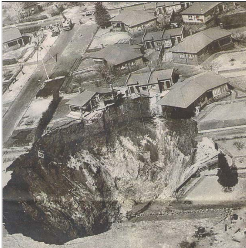
Figure 37: Footage of a sinkhole in the mining town of Blyvooruitzicht, Far West Rand, 1964. Media photograph. (Eybers 2010:14).
