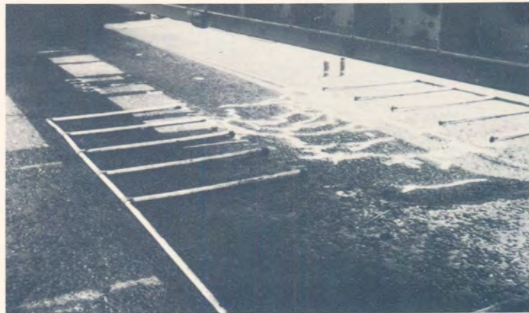
(b) HVS test 1 (215A3): Note the water inlet pipes on the front part of the test section. The white paint indicates the fatigue cracking of the asphalt during the wet test. The uncracked section at the back, is an indication of the surface during dry test conditions. E80s on dry test section: 21 \times 10^6 .
