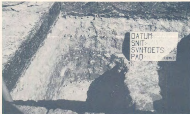
(c) Excavated depth profile of the road structure.
