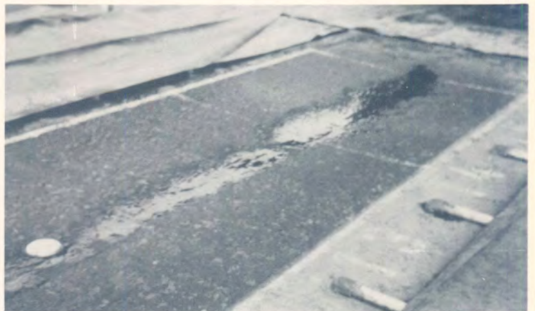
(c) Start of water pumping from the bottom of the crack on SECTION 1.
