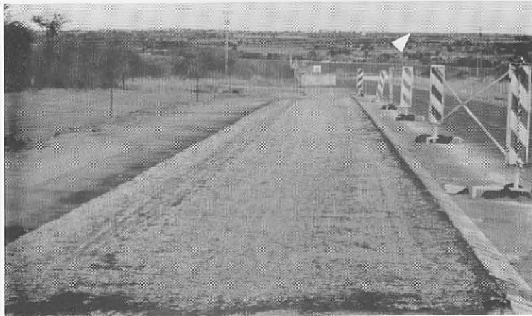
(c) Base layer after the application of the prime coat.
