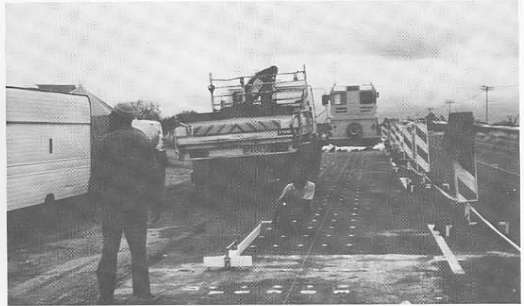
(b) Measurement of surface deflection prior to "crack and seat" operation.
