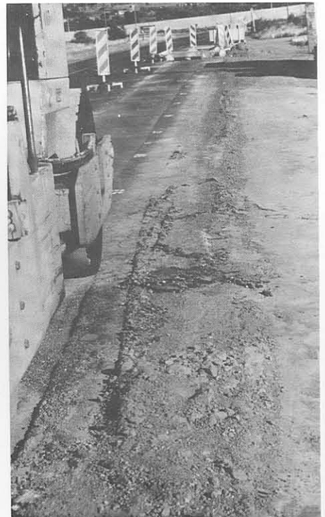
(d) Vibratory roller in operation during the "crack and seat" method.
