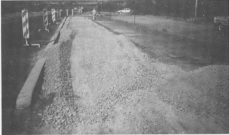
(a) Granular base material on the precracked cemented subbase.
