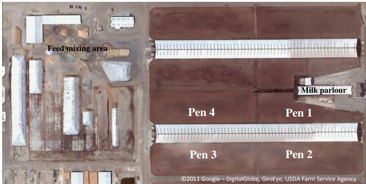
Figure 3.1: Aerial view of the design of Cloverdale South dairy near Hanford, CA, USA.
