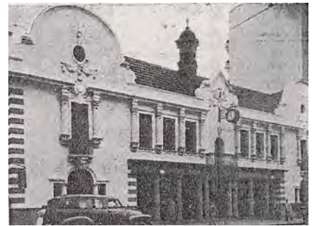
Figure 5: Photograph of the old Town Hall with the City Centre building in the background (Pretoria News, 15 March 1957).
