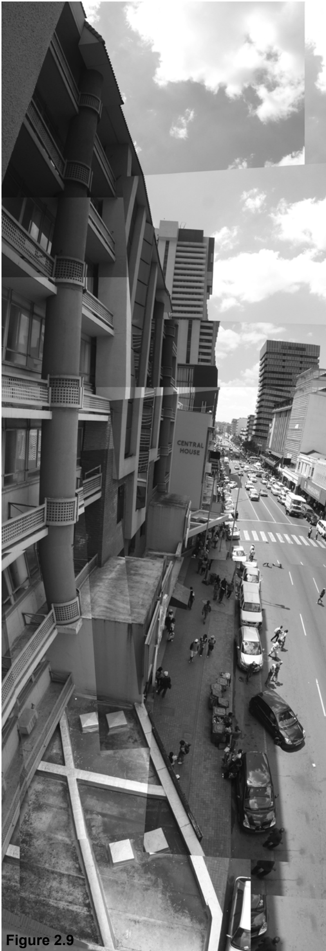
Fig.2.9 - Multirama view of Pretorius Street from Die Meent building empty floor towards the east.
