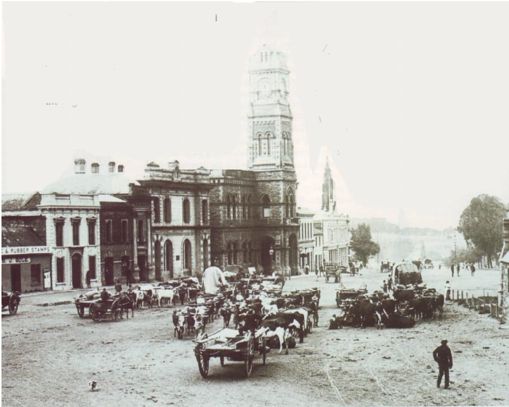
Figure 86: The Town Square Grahamstown 1903 note the ox wagons. Most early South African towns have extremely wide streets to allow a fully spanned ox-wagon to U-turn. (O'Meara:1995:16)
