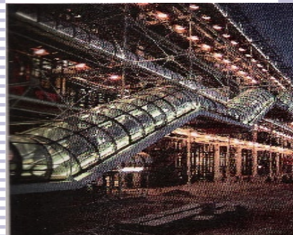
Fig. 146 Pompidou National Centre for Arts and Culture-movement clear. Fleming, W (2001:661) Building by Renzo Piano and Richard Rogers
