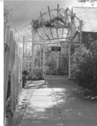
Fig.10 Historic building with poor access
