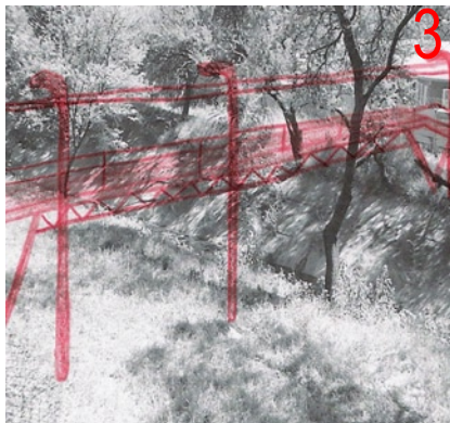
Fig. 27 Bridge crossing the Apies River culvert
