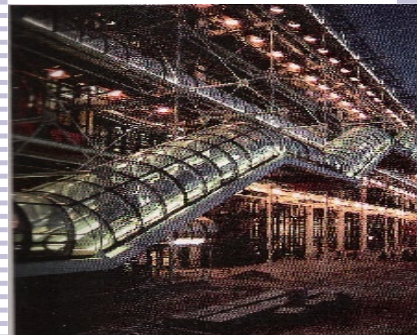
Fig. 146 Pompidou National Centre for Arts and Culture-movement clear. Fleming,W (2001:661) Building by Renzo Piano and Richard Rogers
