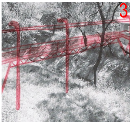
Fig. 27 Bridge crossing the Apies River culvert
