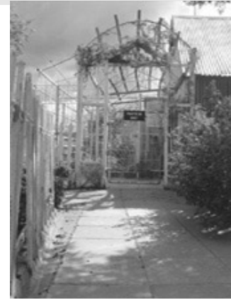
Fig.10 Historic building with poor access
