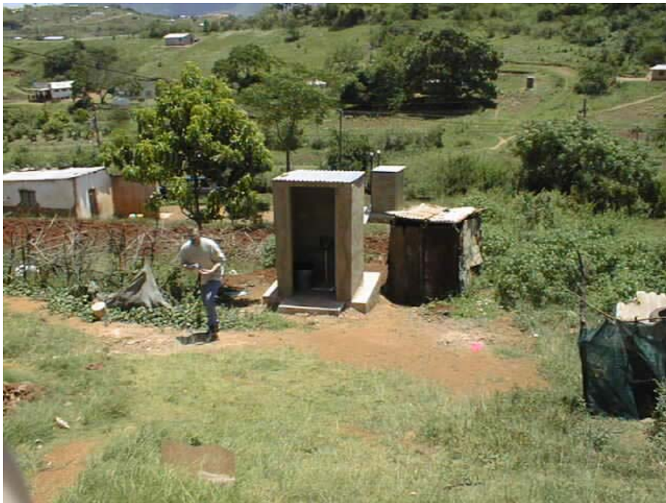
Figure 6.8: Using the natural ground slope to minimise steps at the entrance and depth of vault below ground level (2) (Photographs: F. Stevens, eThekweni Water Services)
