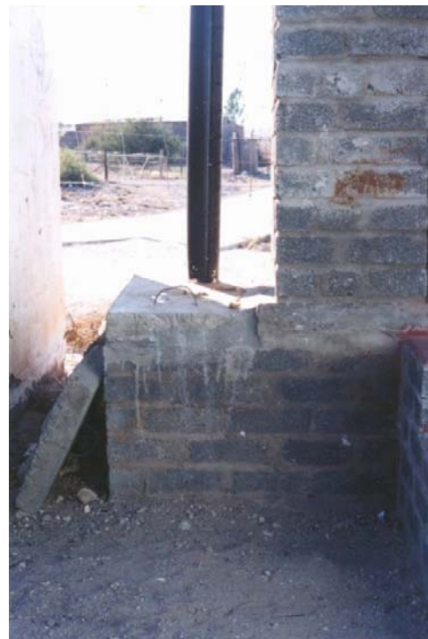
Figure 6.10: Examples of poor practice (1): It is extremely difficult to gain access to these vaults for emptying purposes (Photographs: CSIR)
