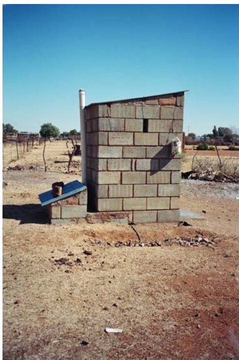
Figure 6.10: Examples of poor practice (1): It is extremely difficult to gain access to these vaults for emptying purposes (Photographs: CSIR)
