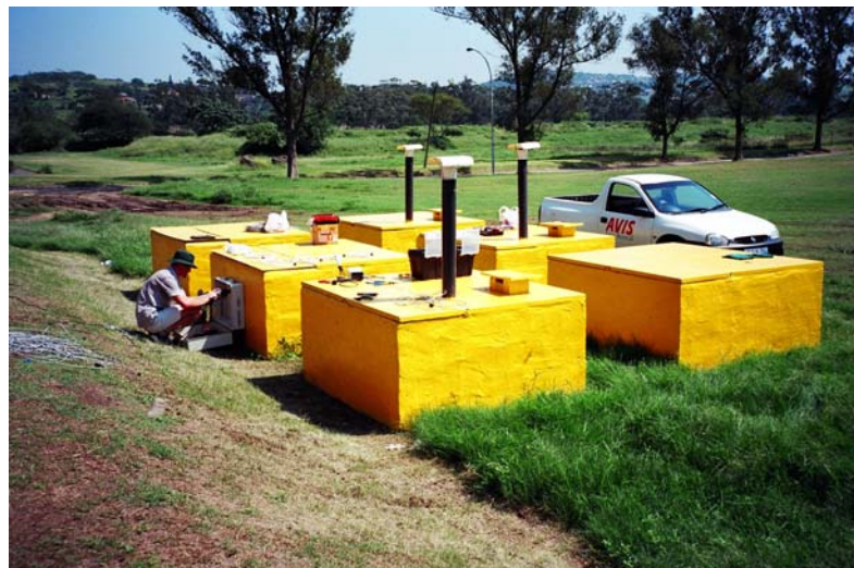
Figure 5.4: Completed vault layout
