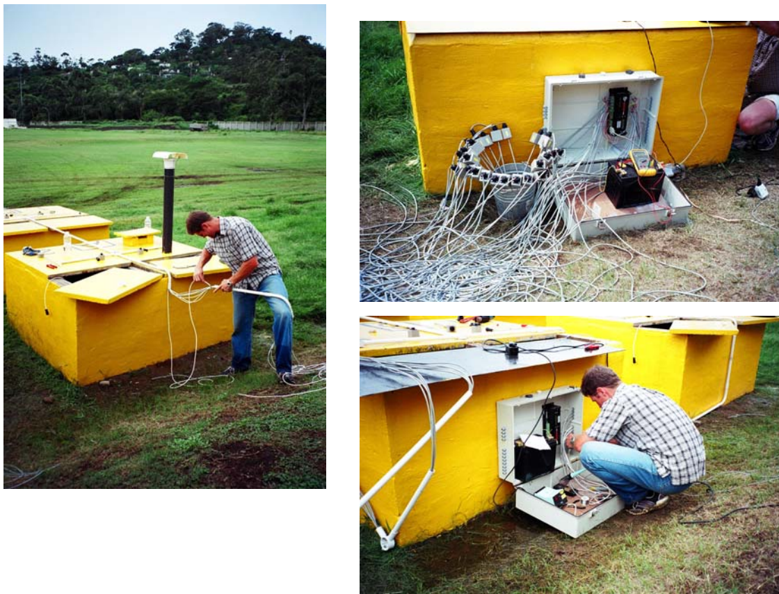
Figure 5.9: Calibrating and installing the temperature probes and data logger
