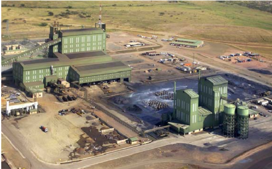
Figure 2 Aerial photograph of the furnace and metal treatment building (upper left hand corner) and slag processing building (lower right hand corner). The block yard is located between these two buildings.
