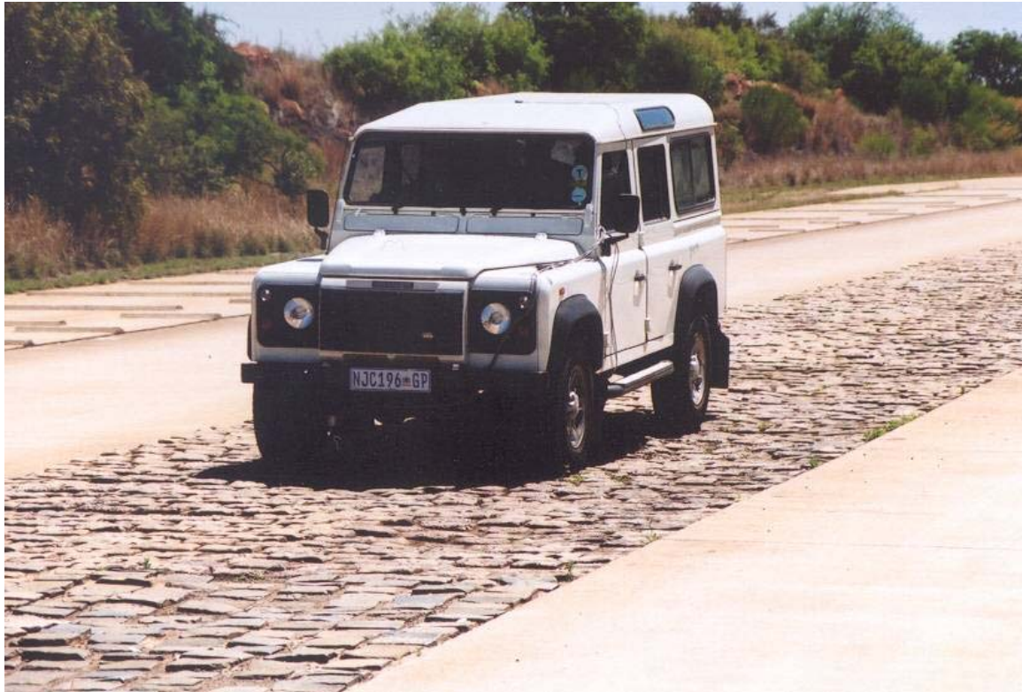
Figure 2.21 - Belgian paving
