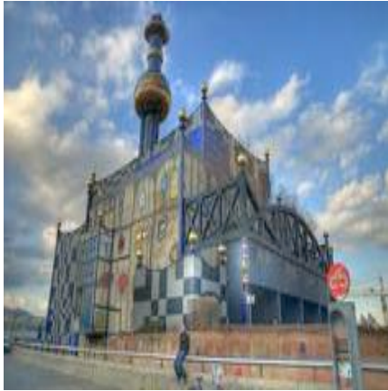
Figure 4.5. Photo V. Durant, 2010 Site Visit and Tour August 2010.
