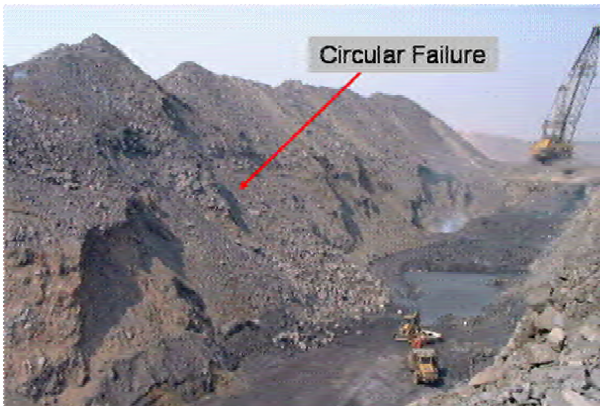
Figure 3.6 - Photo of Circular Failure
