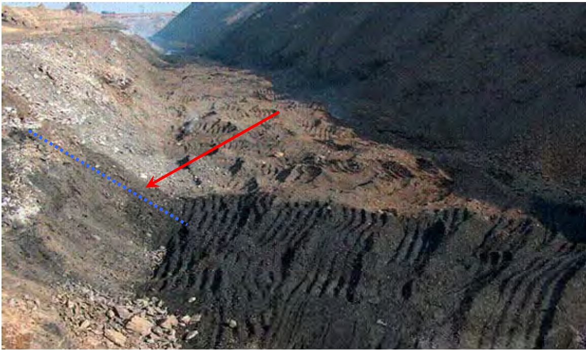
Figure 2.5 - Photo of Highwall post-buffer blasting
