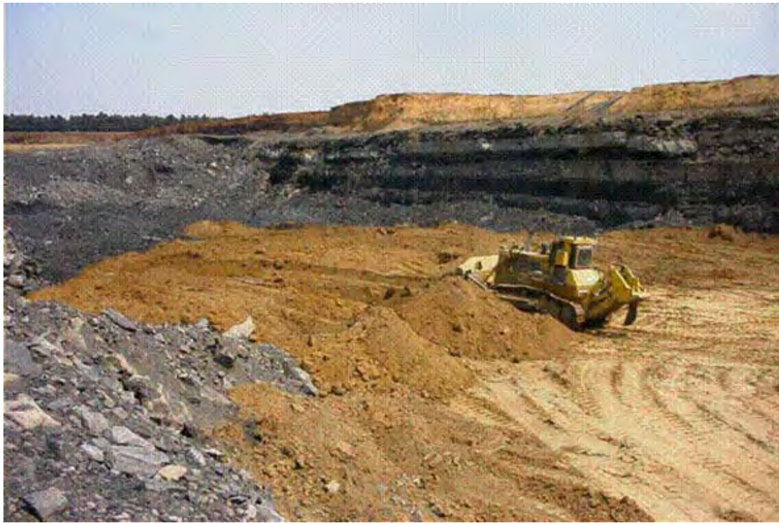
Figure 2.6 - Photo of buffer being cladded
