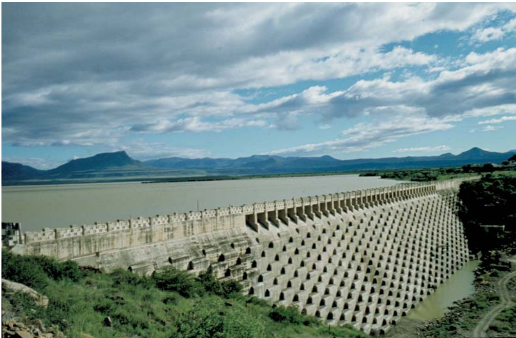
Figure 7.1 - Van Ryneveld's Pass Dam (view from downstream)
