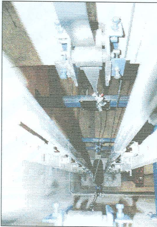
Figure 84 View through the mouth of the shaft.
