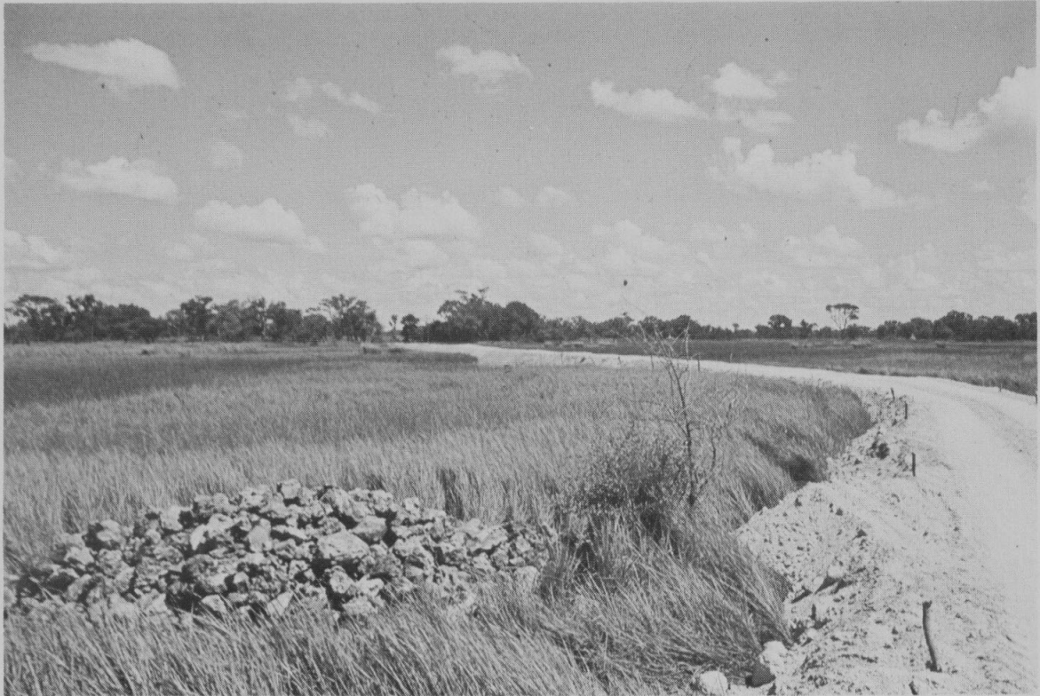
FIGURE 28 – Bunding of Primary Floodplain Communities by Anglo American Corporation offstream of the lower Boro River floodplain system during 1973, Okavango Delta, Botswana.
