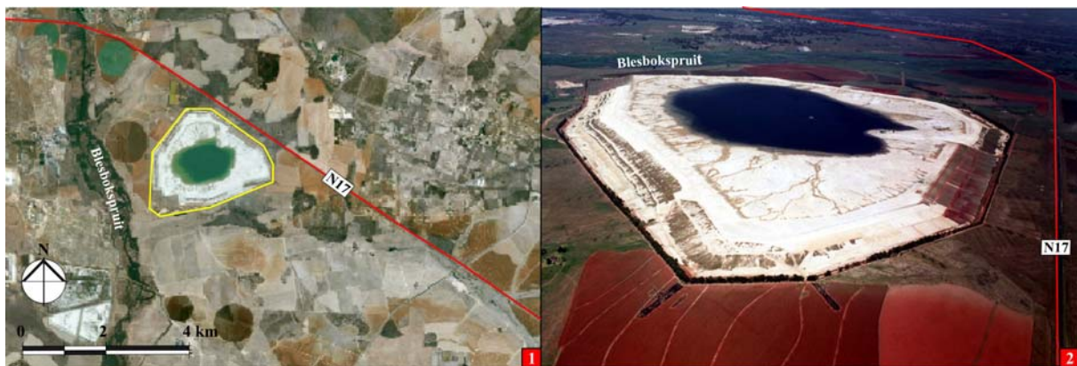
1 Looking north-east over ERGO Daggafontein tailings impoundment.
