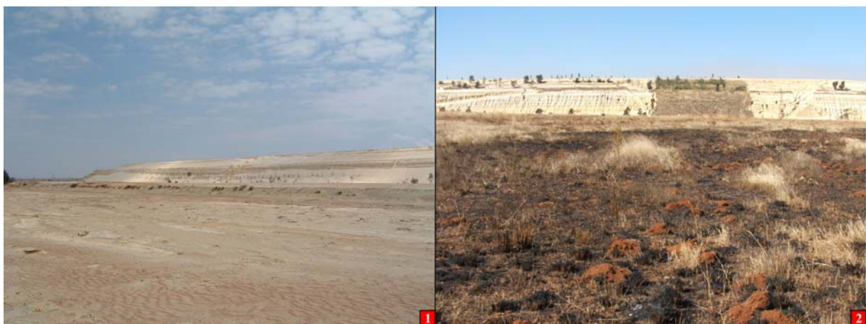
1 Looking north-west towards the southern slope of the south-western compartment of the DRD 2L24 tailings impoundment.
