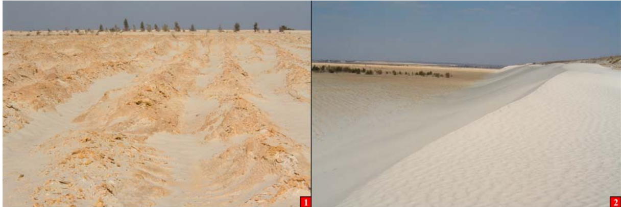
1 Looking East over a section on the top surface of the DRD 2L24 tailings impoundment which had been ridge ploughed.
