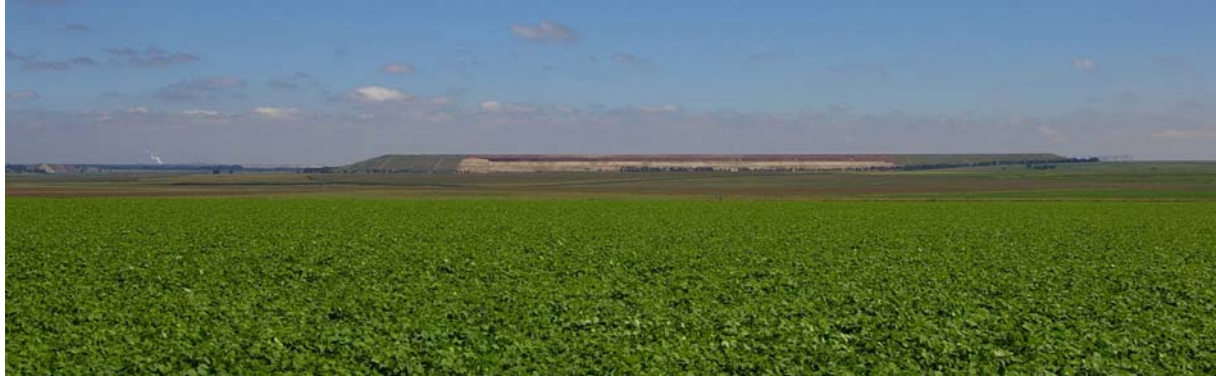
Figure 87: The ERGO Daggafontein tailings impoundment lies within an area with a rural character and rolling topography.
