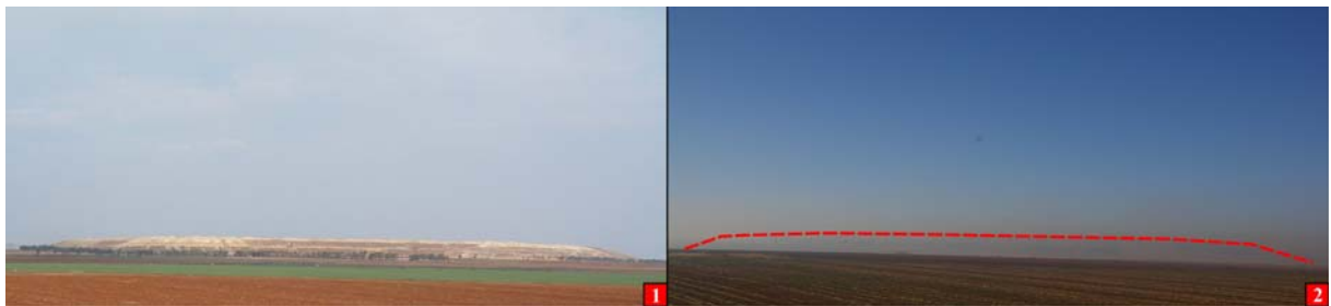
Figure 104: Looking south-east towards the ERGO Daggafontein tailings impoundment.
