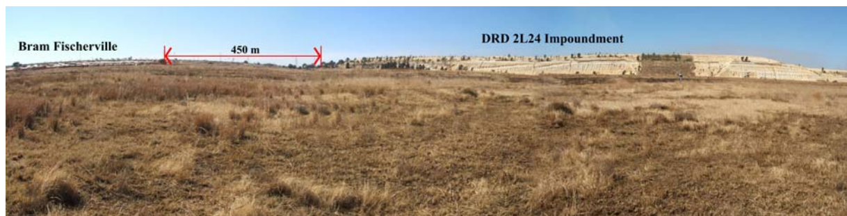
Figure 117: Current and proposed extensions of Bram Fischerville adjacent to the DRD 2L24 impoundment.
