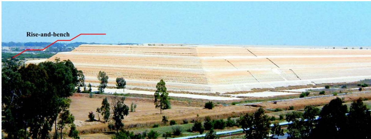
Figure 74: Typical side slope profile of an upstream constructed ring-dyke gold tailings impoundment.
