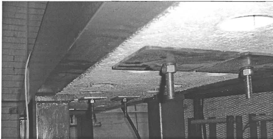
Figure A.17 Concrete reinforcing of the test bench
