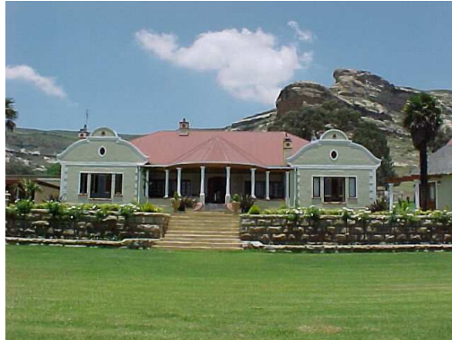
FIGURE 4.2: THE GUEST HOUSE SITUATED ON ORANJE FARM
