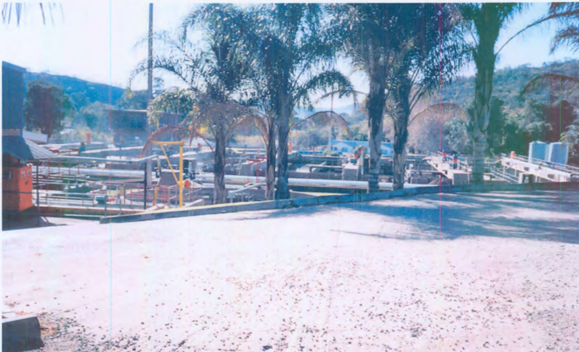
Figure 5: Daspoort Wastewater Treatment Works
