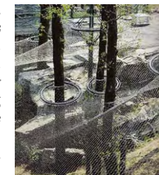
Figure 110. Burger's Zoo, Arnhem. The Netherlands Leopard and jackal enclosures. Stainless steel cable net. Artificial trees are used for support to help the existing oak trees support the enclosure. (p111,114) (photo by Hans George Esch, Germany)
