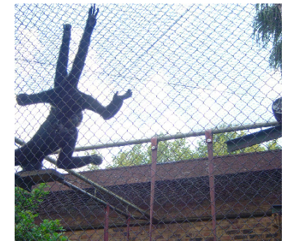
Figure 25. Gibbon Enclosure, SA Zoo. Volumetric linear elements are used for animals to walk on and to play on (structural steel skeleton and wire mesh).
