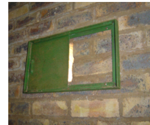
Figure 127. Access to breeding boxes from the existing Service Passage.
