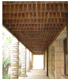
Figure 81. Wooden walkways are supported by solid construction.
