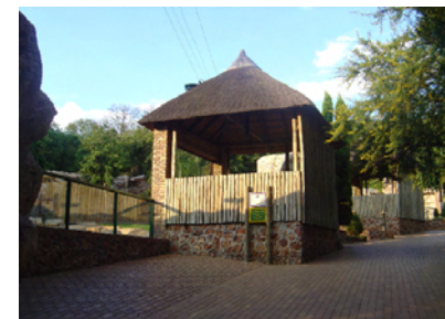
Figure 40. Viewing structures of the Bear Enclosure, SA Zoo. Three covered viewing structures are repeated along the main path in a linear organization, for visitors to recess in these spaces while watching the animals at a different height.
