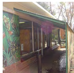
Figure 82. A covered walkway at the Snake Enclosure.
