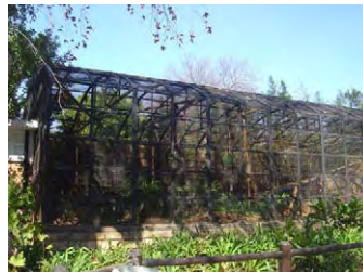
Figure 68. Steel supports forming the skeleton of enclosures.
