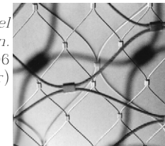
Figure 109. A balustrade of X-tend mesh, Germany. X-tend offers transparency.
