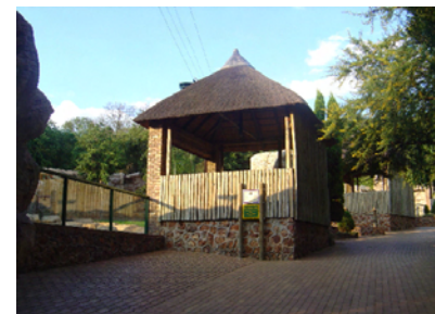
Figure 40. Viewing structures of the Bear Enclosure, SA Zoo. Three covered viewing structures are repeated along the main path in a linear organization, for visitors to recess in these spaces while watching the animals at a different height.
