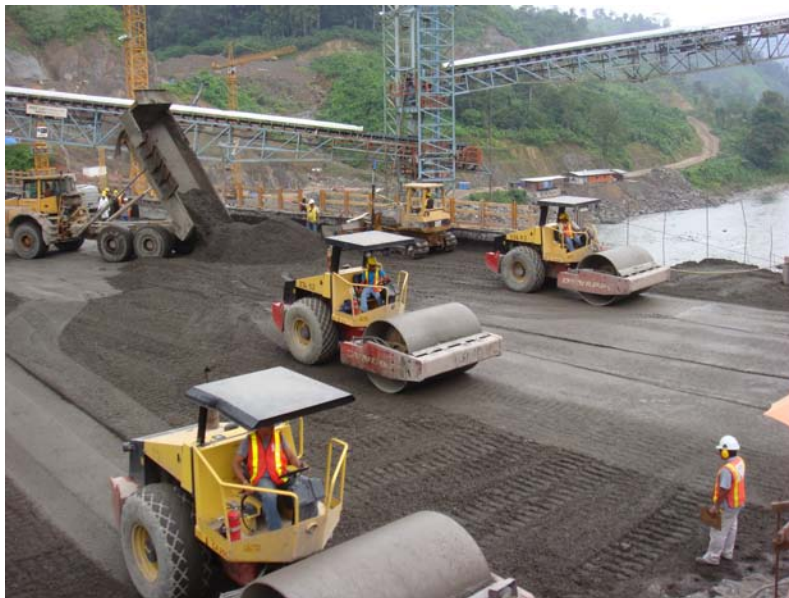
Plate 2.2: RCC Compaction
