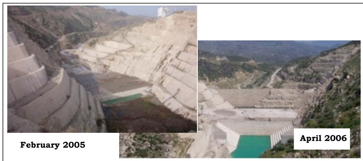
Figure 2.8: Çine Dam Construction Progress
