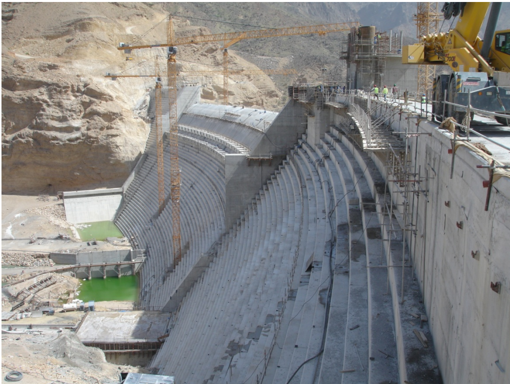
Plate 4.5: Wadi Dayqah Dam – May 2009
