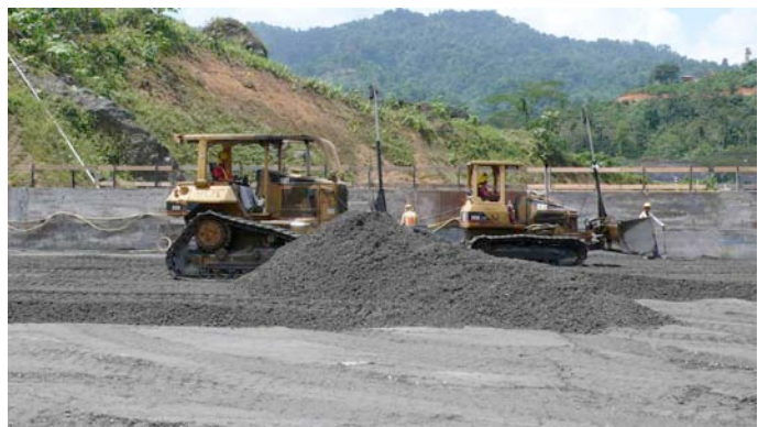
Plate 5.4: RCC Placement at Changuinola 1
