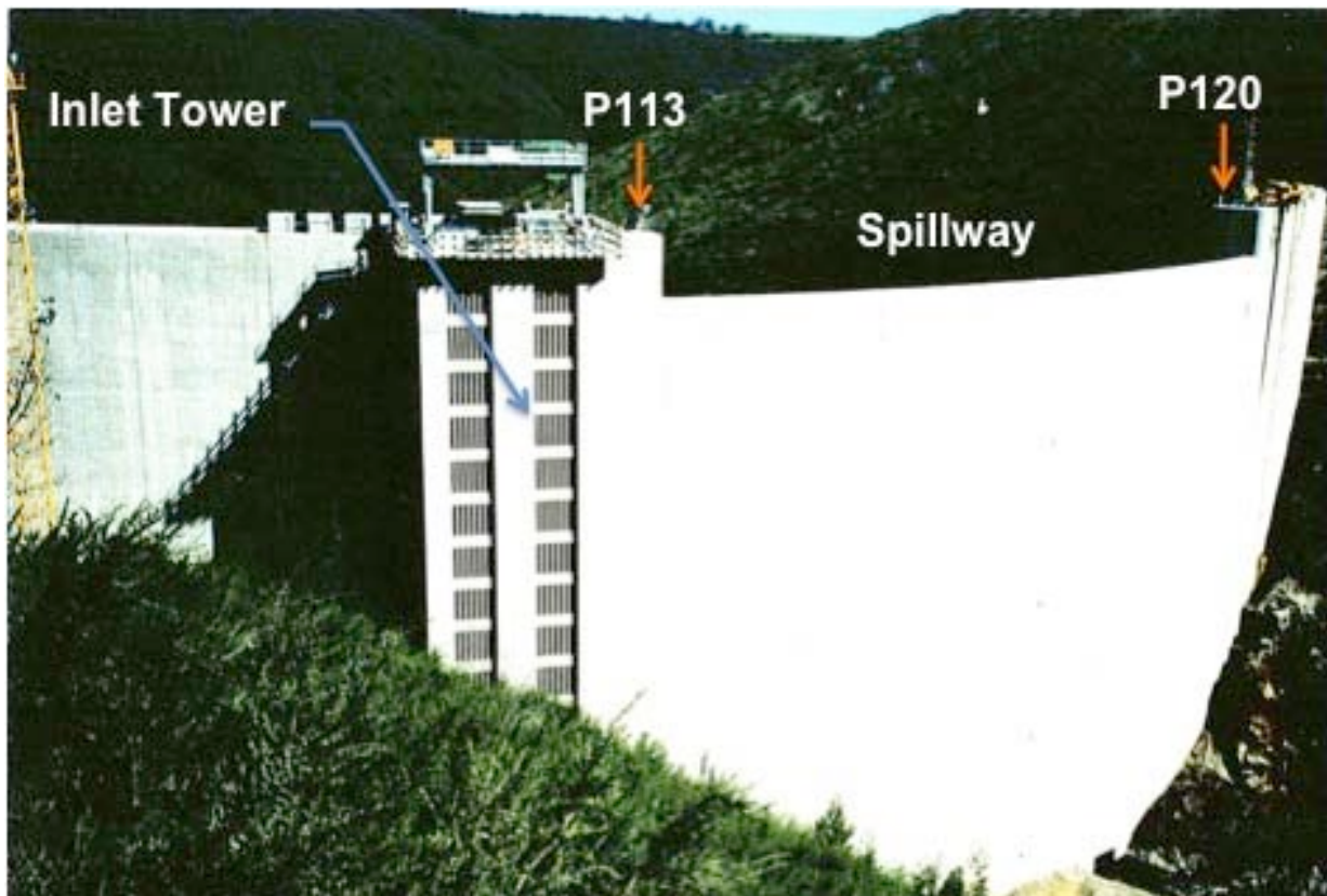
Plate 5.3: Upstream View of Dam Illustrating Beacons, Tower & Spillway
