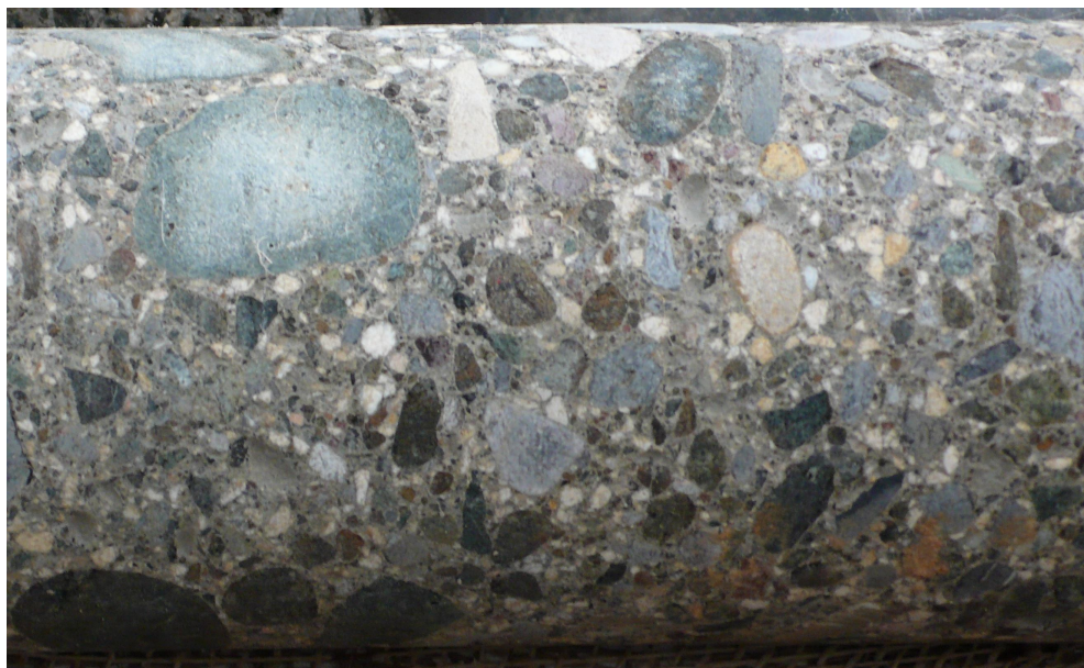
Plate 6.3: Typical Modern High-Paste RCC
