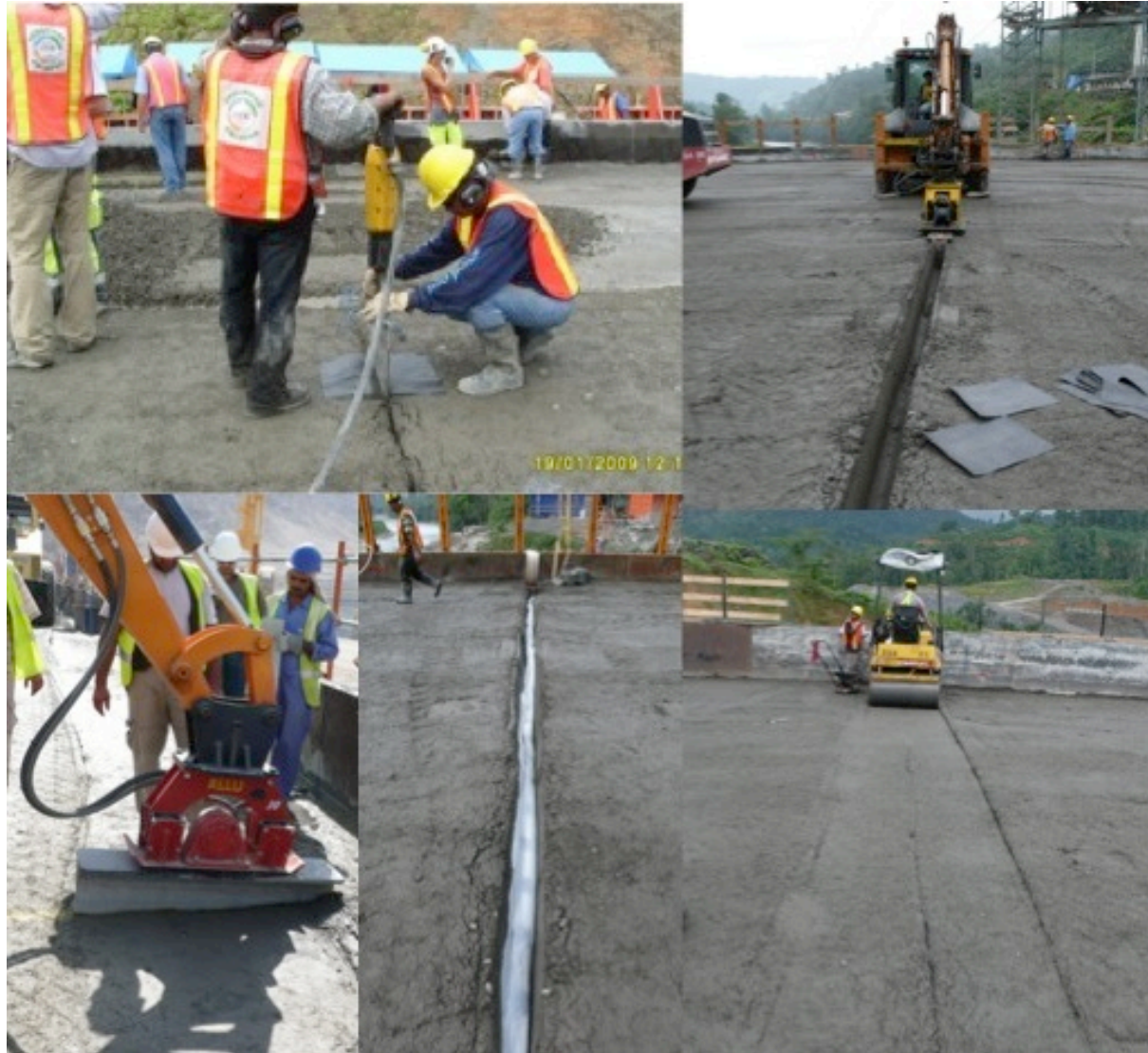
Plate 2.5: Induced Joint Inserted into Compacted RCC
