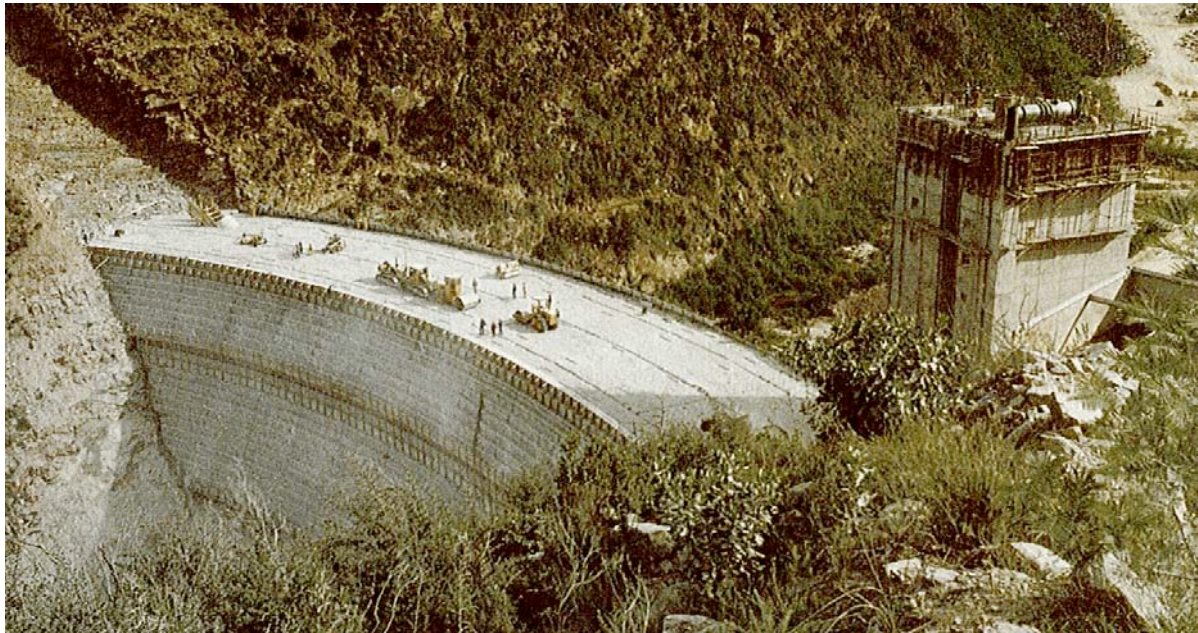
Plate 5.1: Wolwedans Dam Instrumentation Installation at RL 66.25 m
