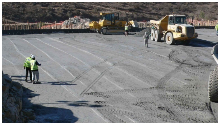
Plate 3.2: A Modern RCC at De Hoop Dam
