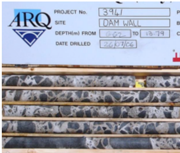
Plate 6.1: Typical Low Grade Dam Mass Concrete (1950s)
