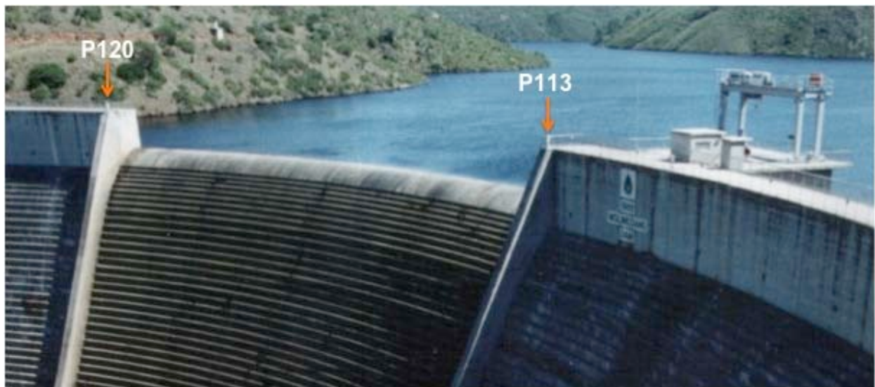
Plate 5.2: Wolwedans Dam – Illustrating Crest Beacons P113 & P120
