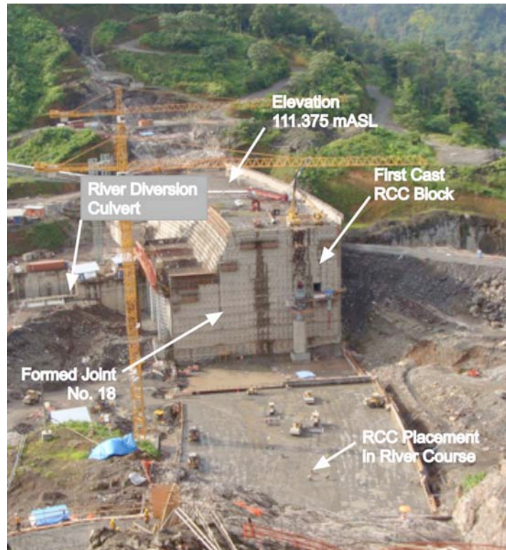
Plate 5.5: RCC Placement at Changuinola 1
