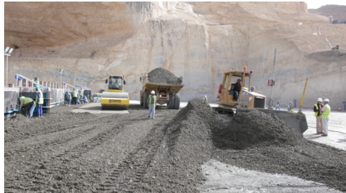
Plate 4.4: Early RCC Placement
