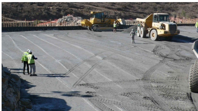
Plate 3.2: A Modern RCC at De Hoop Dam
