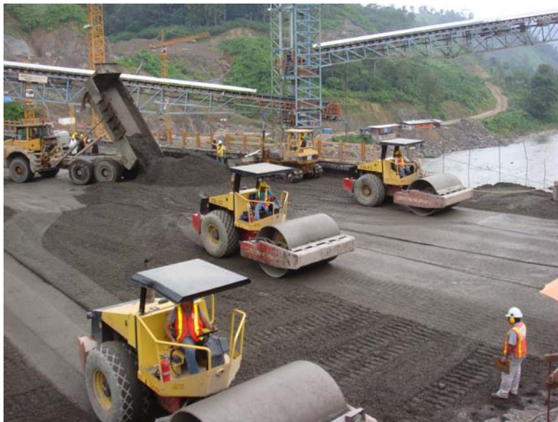
Plate 2.2: RCC Compaction
