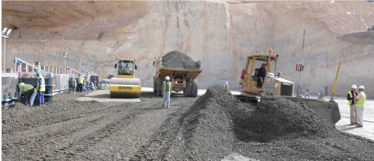
Plate 2.1: RCC Construction- Dumping, Spreading & Compaction
