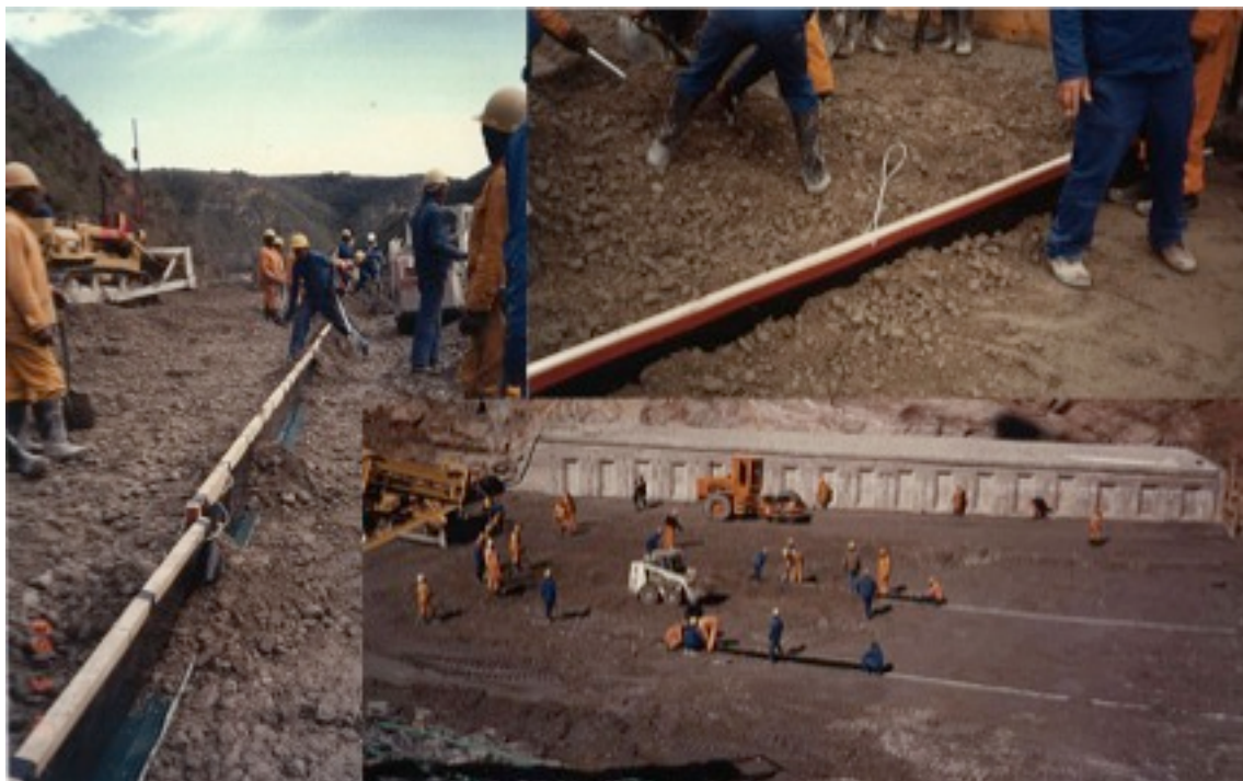
Plate 2.4: Induced Joints Inserted into RCC with Placement (3)
