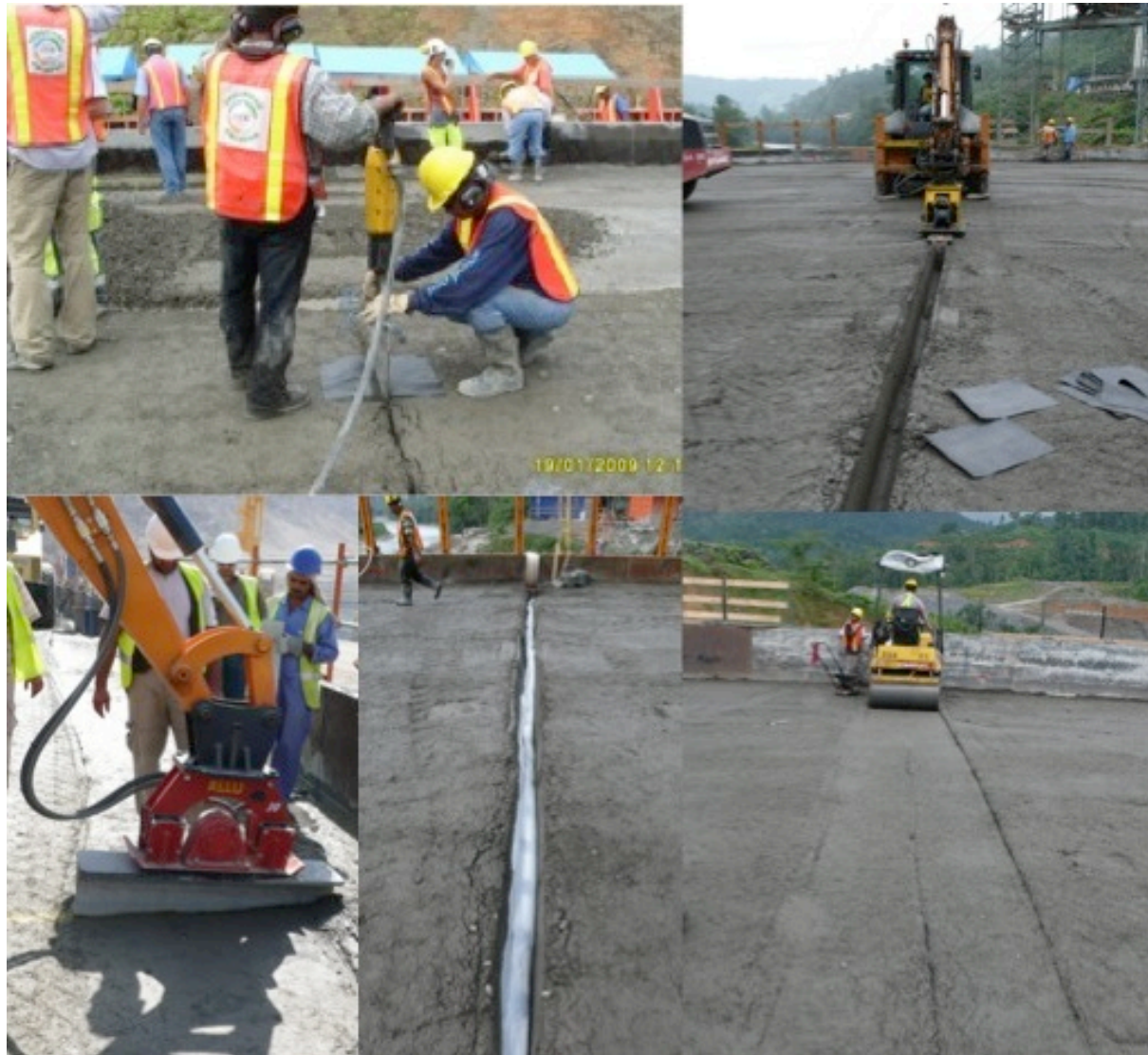
Plate 2.5: Induced Joint Inserted into Compacted RCC
