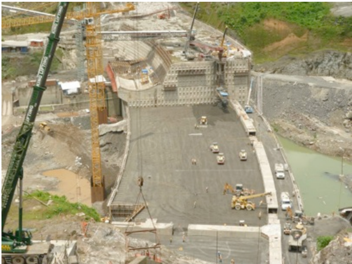
Plate 2.16: Construction Progress at Changuinola 1 Dam on 25 th June 2010
