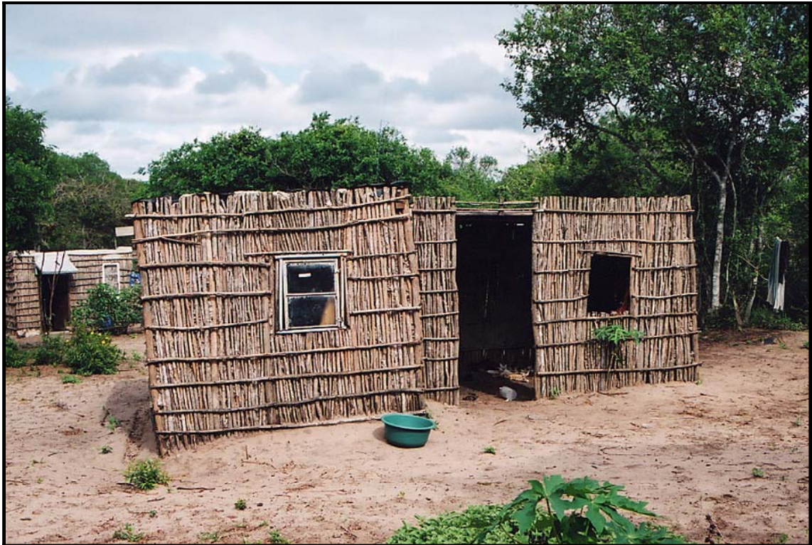
Figure 6: A complete house with several rooms. This house consists of two bedrooms (one of them visible to the left with a glass window) separated by a common room to which is attached an unclosed veranda style room to the right that also serves as a kitchen. The walls are made entirely of small wooden poles stacked between larger supporting poles. The roof consists of corrugated iron sheets supported by wooden beams. Note the single room house in the background to the left, built in the same style. Photo by J. Gaugris: Manqakulane community, northern Maputaland, KwaZulu-Natal, South Africa, 2002.
