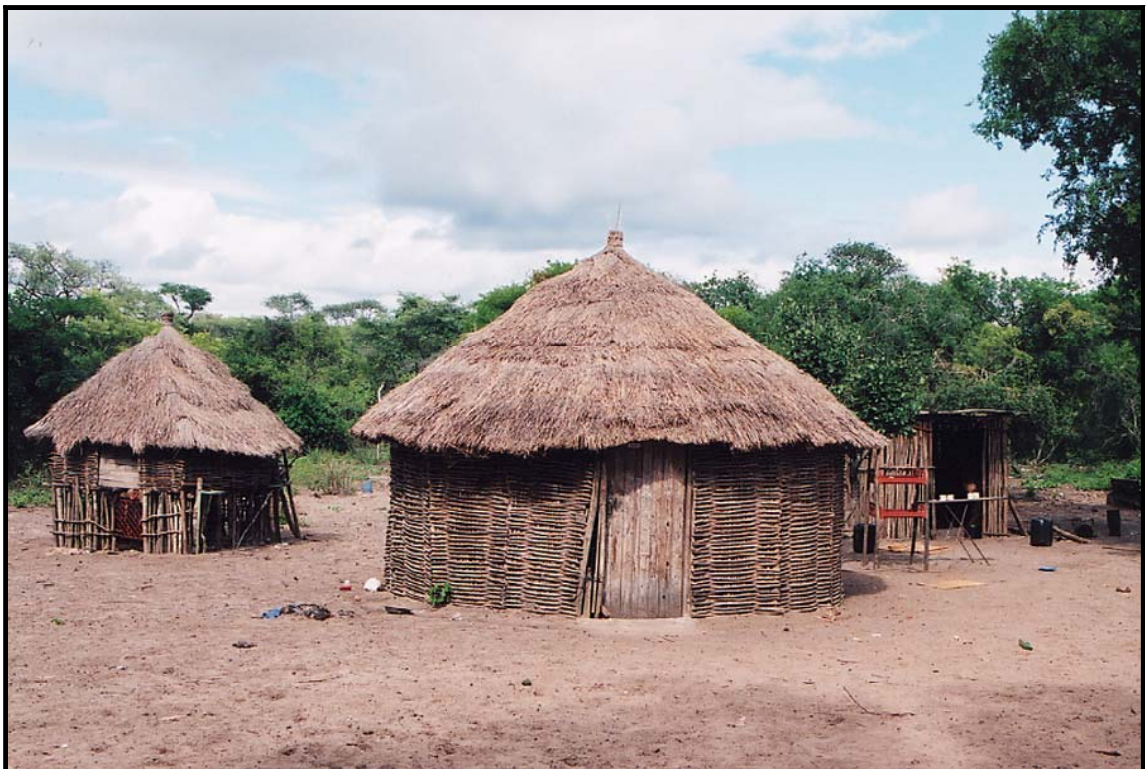
Figure 7: A single room round house (middle), flanked by a maize store raised on a platform (left) and a kitchen (right). The walls of the house and maize store are made of a wooden lattice stacked between larger supporting poles. The kitchen walls are made of planks. The roofs of the house and maize store are thatched while the roof of the kitchen consists of corrugated iron sheets supported by wooden beams. Note the chicken pen under the maize store. Photo by J. Gaugris: Manqakulane community, northern Maputaland, KwaZulu-Natal, South Africa, 2002.
