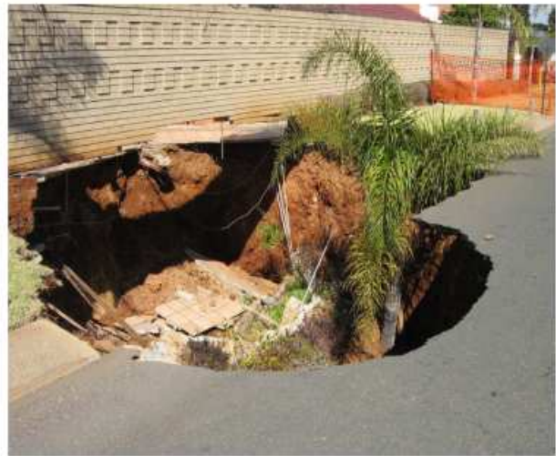
Figure 10a: Sinkhole in Laudium corner 7 th Avenue and Pendant street measuring 20 m x 10 m in dimension (July, 2007.)
