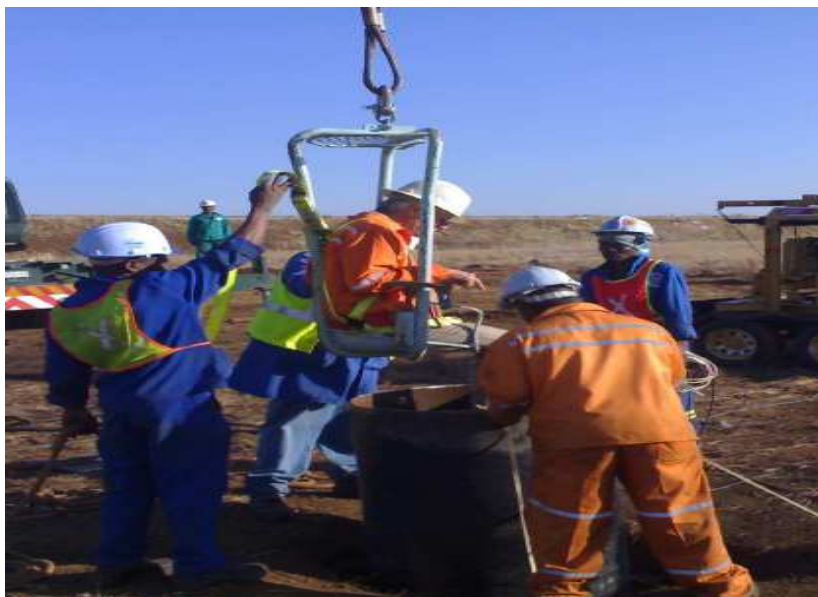
Figure 21: An engineering geologist being lowered down a hole for profiling
