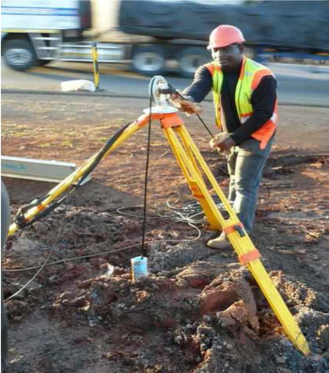
Figure 15: Borehole radar survey at pier location
