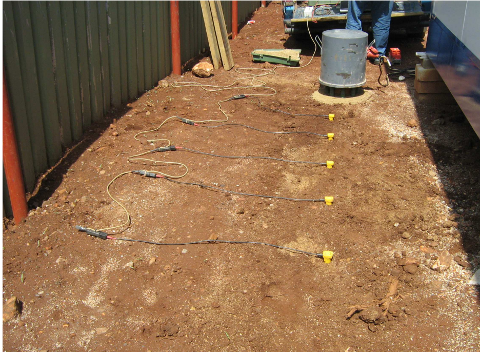
Figure 19: Continuous Surface Wave testing showing geophones and a shaker
