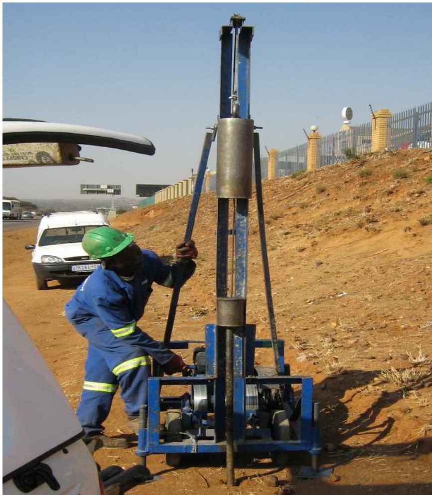
Figure 24: Dynamic Probe Super Heavy testing in Techno Park
