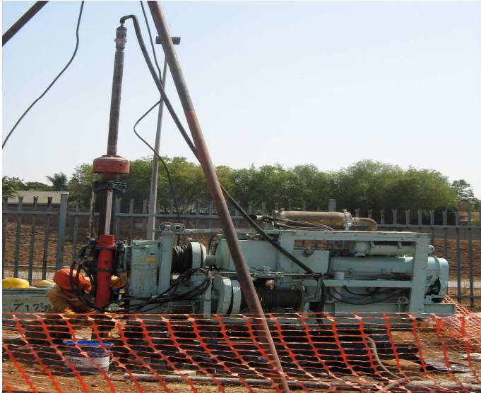
Figure 13: General view of a Rotary Core drilling rig
