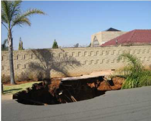
Figure 10a: Sinkhole in Laudium corner 7 th Avenue and Pendant street measuring 20 m x 10 m in dimension (July, 2007.)
