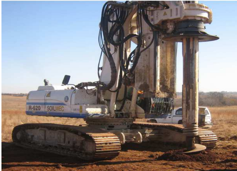
Figure 20: Large Diameter Auger Rig drilling in the Military area
