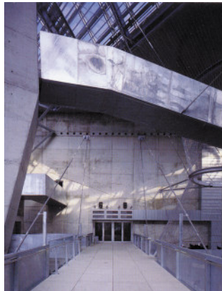
Fig 56. Bridge enclosed by galvanized metal balustrades
