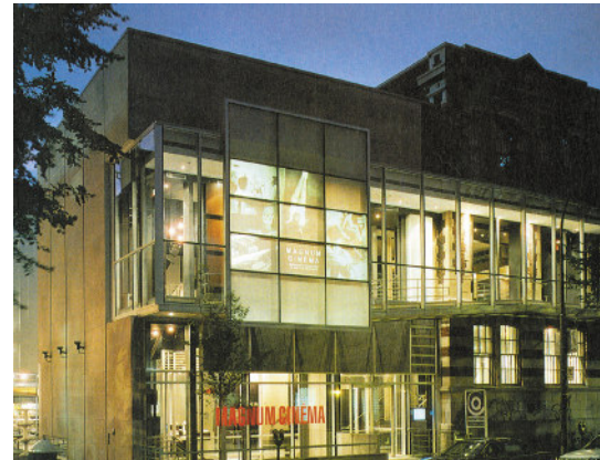
Fig 36. Glass facade and translucent screen
