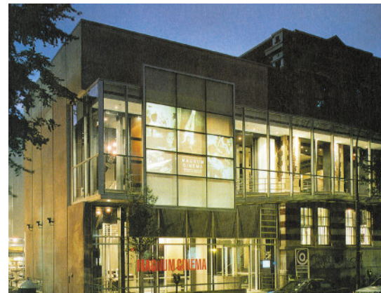
Fig 36. Glass facade and translucent screen
