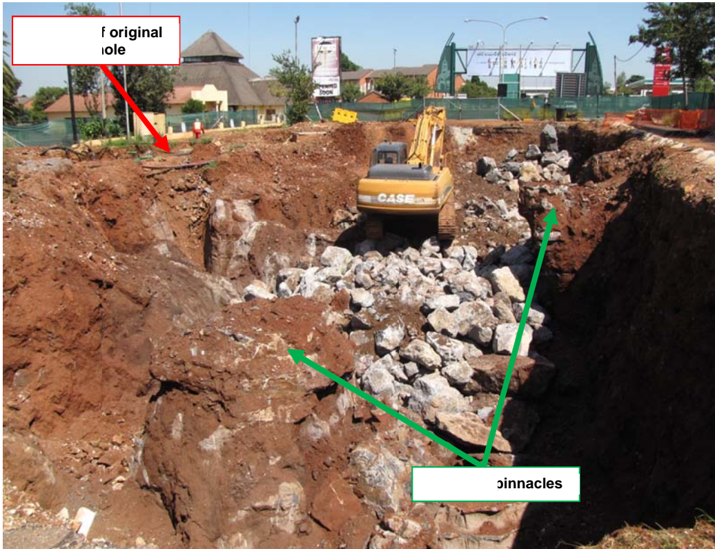
Plate 21. Remediation of the sinkhole Jean Avenue (S109)
