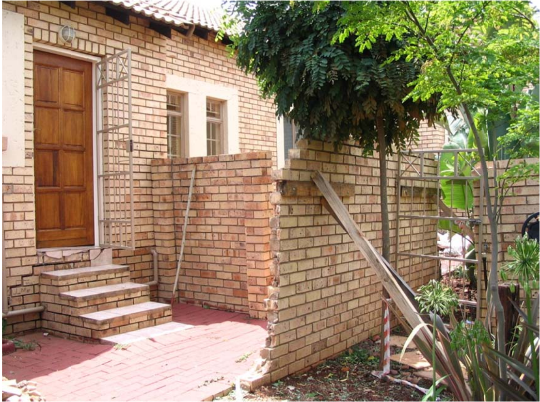
Plate 17. A settlement in a residential complex, Die Hoewes (S97)
