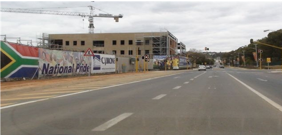
On the barriers of a building site
