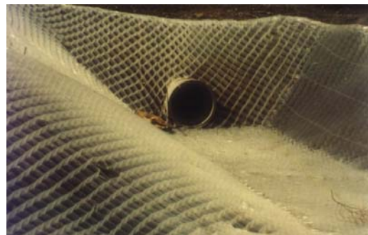
d) Geocell for storm water channel lining.
