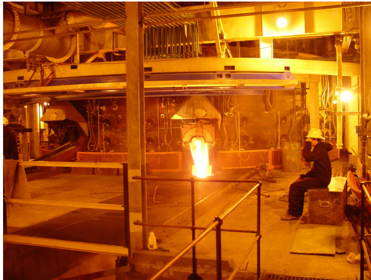
Figure 30: Tapping slag from the slag cleaning furnace. Photograph taken by R. Hundermark and displayed courtesy of Rustenburg Platinum Mines Ltd, Waterval Smelter.
