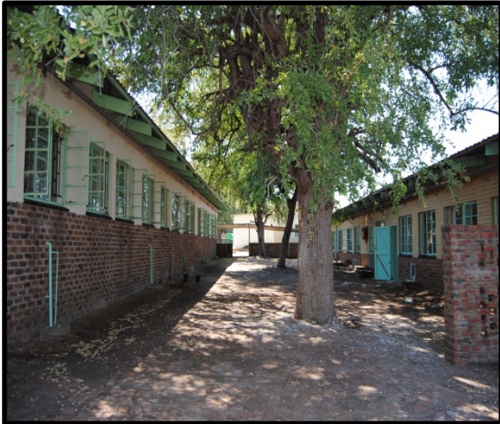
The outside of the ward
