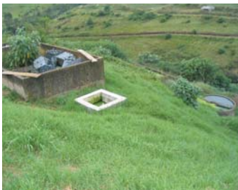
Dairy waste is first filtered through a fat trap before entering the main system.
